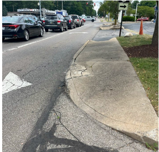
Existing Image 2: Damaged sidewalk on East Market St approaching the Niles Cortland Rd intersection
