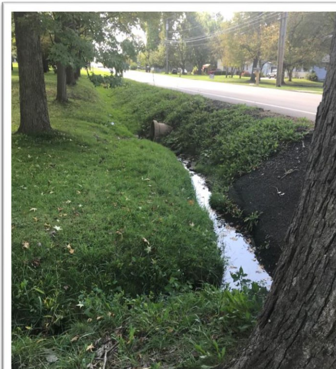
Figure 17 Open Ditches and Culverts
